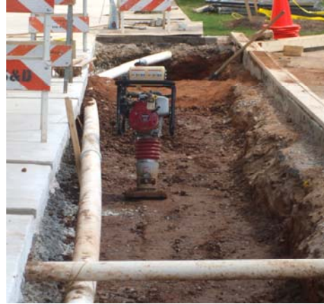
Figure 4. Installation showing individually compacted "lifts".
